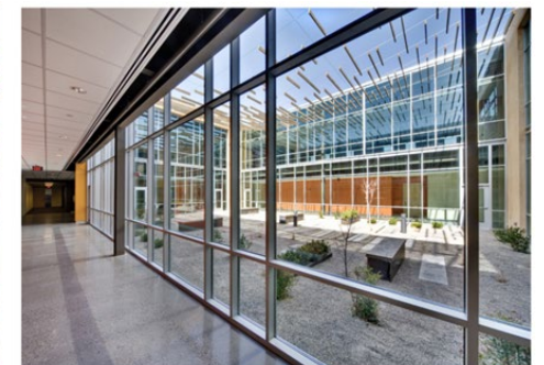
Curtain wall surround the interior courtyard at GSA Office Building (2019) in New Mexico, designed by Page Southerland Page
