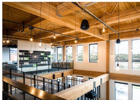
Exposed glulam timber structural beams at 38 Davis building (2016) in Portland, designed by Ankrom Moisan Architects
