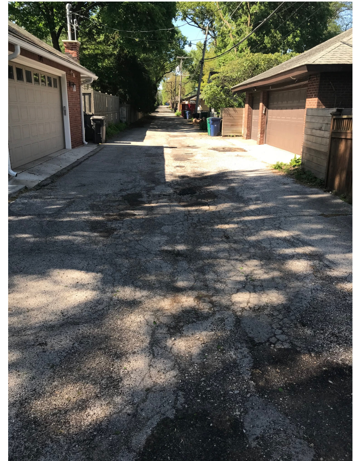
Current Alley Condition
