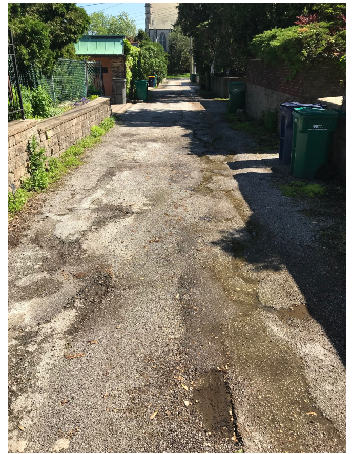
Current Alley Condition
