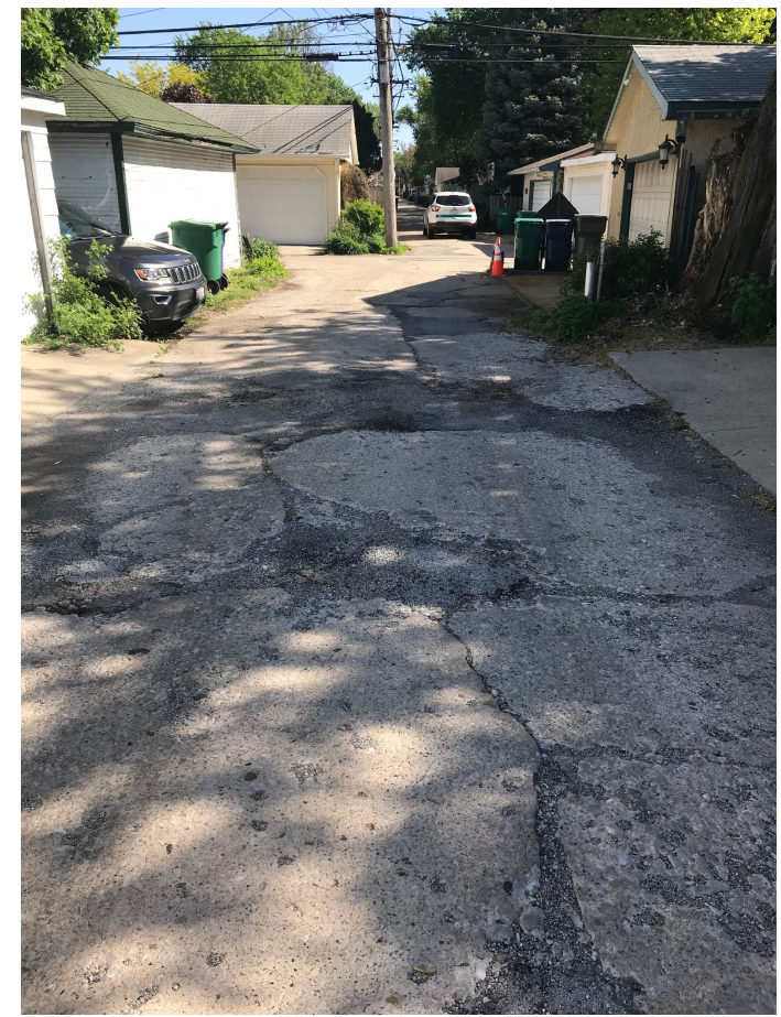
Current Alley Condition
