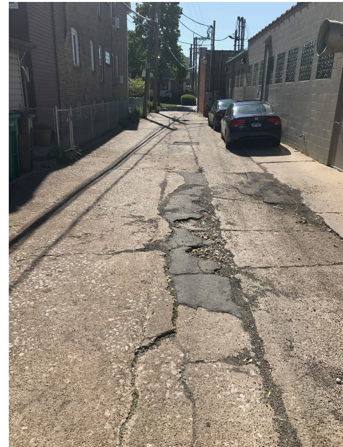
Current Alley Condition
