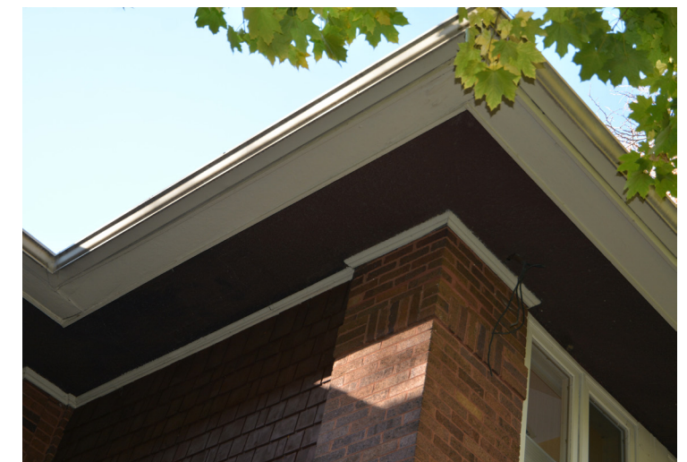
ENLARGED PHOTO OF EXISTING PAINTED CEDAR SHINGLES
