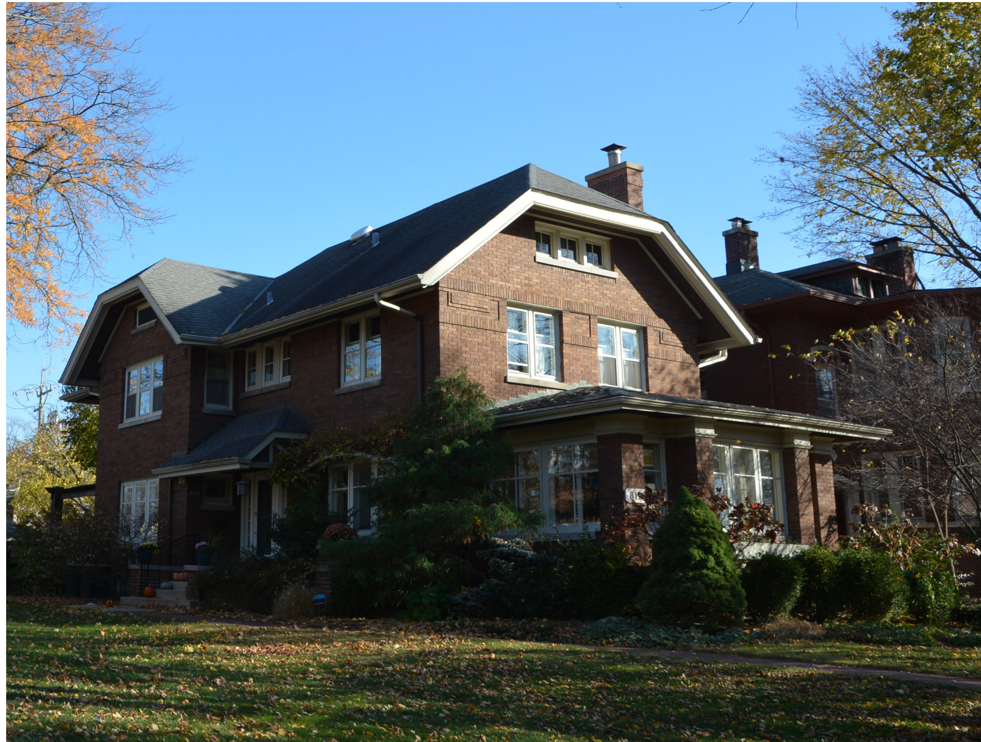
EXISTING RESIDENCE NORTH & WEST FACADES
