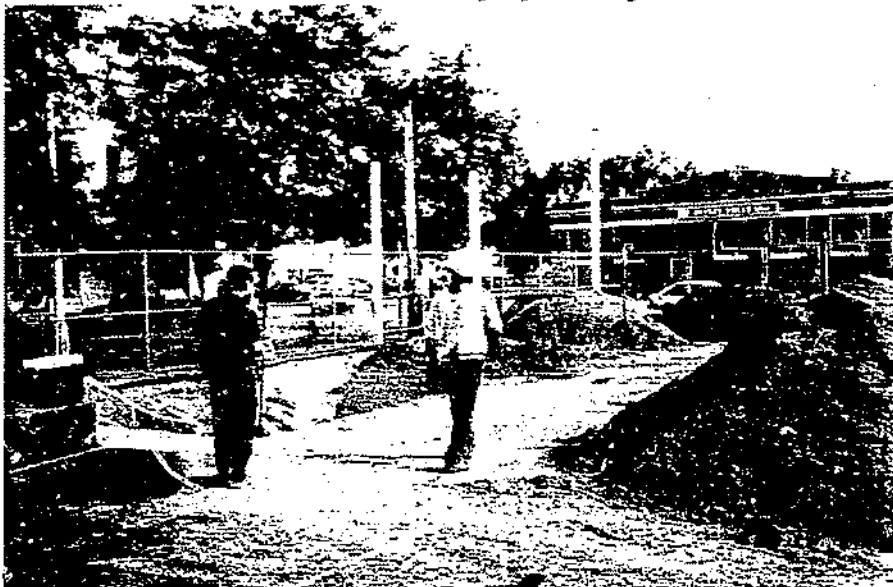
Project Site Facing South
