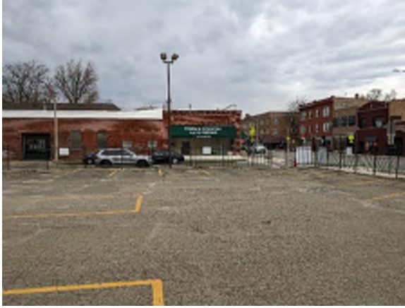
Northeast corner of property facing West
