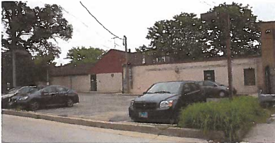
NORTH FACADE - LOOKING EAST
