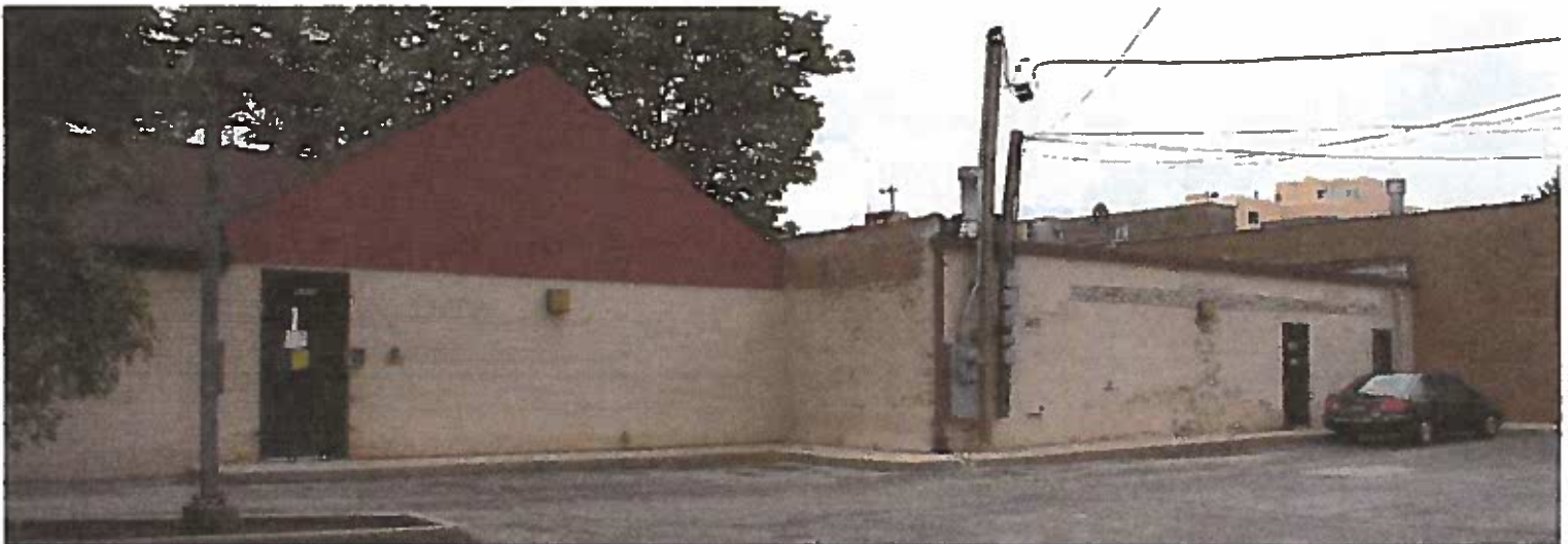
NORTH FACADE - LOOKING WEST
