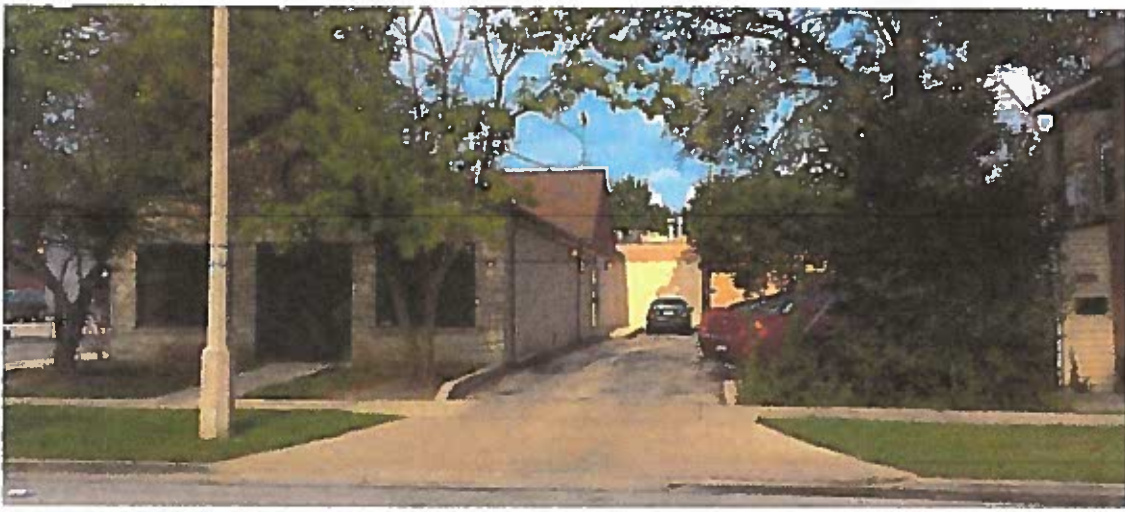
NORTH AND EAST FACADES - LOOKING WEST
