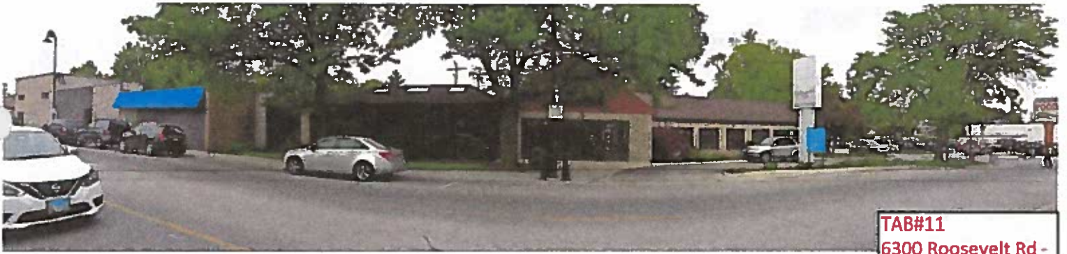
ROOSEVELT FACADE - OVERALL
