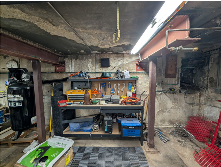
INSUFFICIENT WORK AREA / STRUCTURAL CONSTRAINTS
