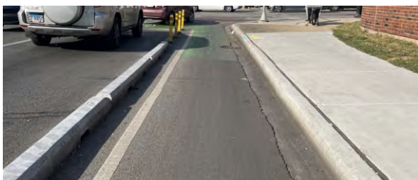
Example of pre-cast concrete curbs
