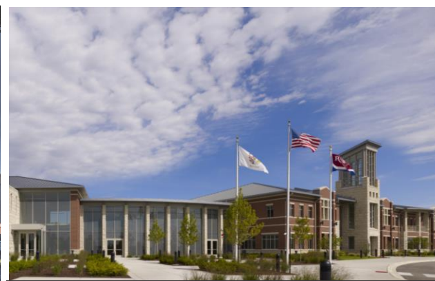
ROMEOVILLE, IL VILLAGE HALL AND POLICE HQ
