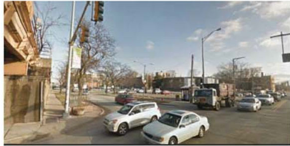
Harlem and South Boulevard - Looking southeast
