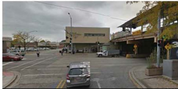
CTA Green Line Entrance at Harlem Avenue
