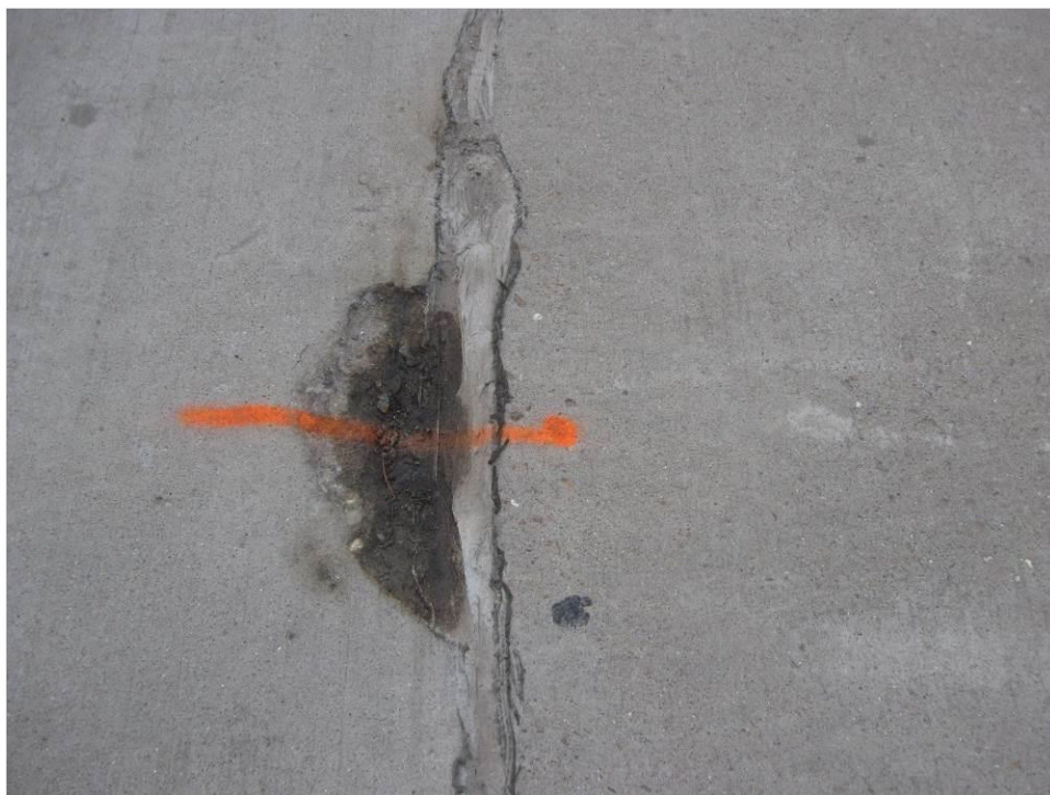
Photo 4 – typical floor spall over shear connector.
