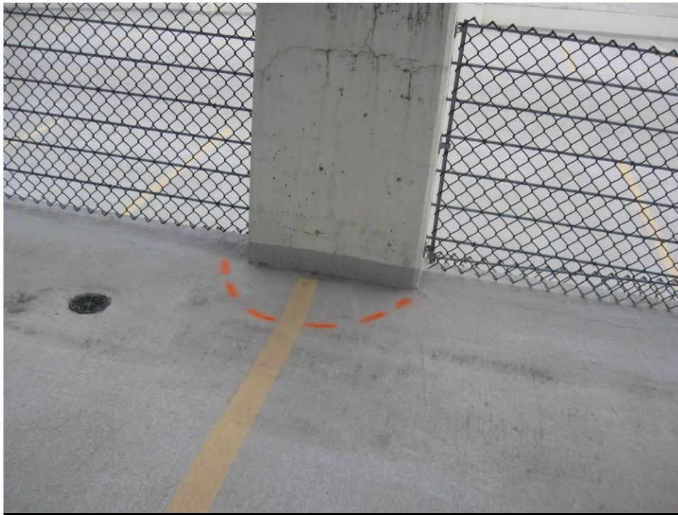
Photo 1 – Typical concrete delamination on floor slabs over top of post-tensioned beams.
