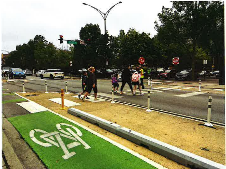
A concrete-protected bike lane and paint and post bumpout on Augusta Boulevard. – 2023 installation
