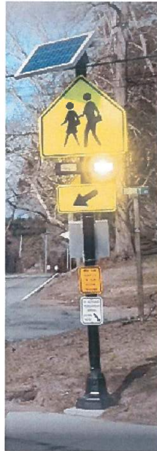
Example of RRFB (Rapid Rectangular Flashing Beacon)
