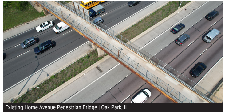
Existing Home Avenue Pedestrian Bridge | Oak Park, IL
