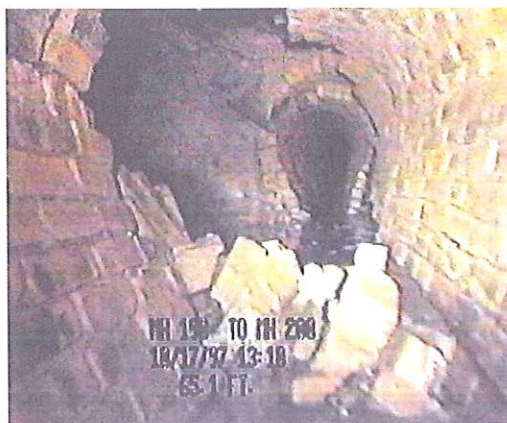
Figure 5. Example of Condition Grade 5 Brick Sewer- Collapsed or Collapse Imminent
