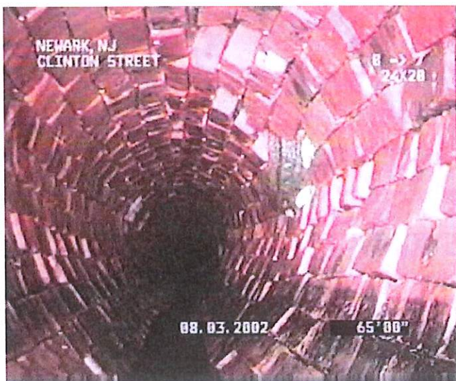
Figure 3. Example of Condition Grade 3 Brick Collapse Unlikely in Immediate Future; Further Deterioration Likely
