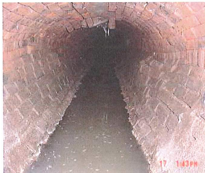
Figure 4. Example of Condition Grade 4 Brick Sewer - Sewer- Collapse Likely in Foreseeable Future
