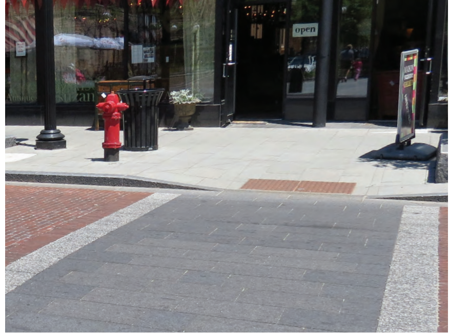
Stone Crosswalk: Thermal cut granite, Oxford Black and Rockville White
