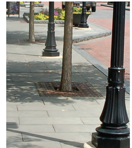
Tree Grate: Garland design by East Jordan, 4'x6' - final size to be determined
