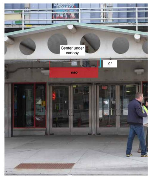
New sign panels and support structure. Sign mounts to existing canopy / beam. Coordinate mounting with existing structure and existing conduit. 90" minimum to bottom of sign from sidewalk.
