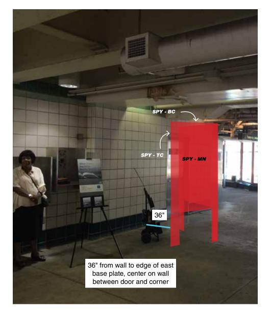
Reuse existing SPY-1.3 structure. Structure will require new CWS snap frames installed in place of existing CWN cabinets. Coordinate with RTA to obtain SPY-1.3 structure. Sign is located in CTA portion of station. Sign is positioned so anchors do not hit concrete seams. Size: 44" x 82" (each side)
