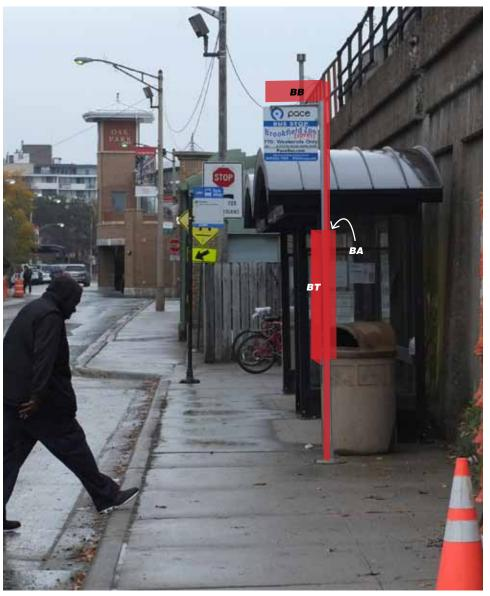
New sign panels, cabinets, sign post, and base replace existing sign post and base. Save existing Pace bus stop sign and mounting hardware. Reinstall existing Pace bus stop sign on new post, using existing mounting hardware. Coordinate existing bus stop sign mounting hardware with new post. Existing CTA route 90-SB sign location (end of line, no boarding) to remain where
