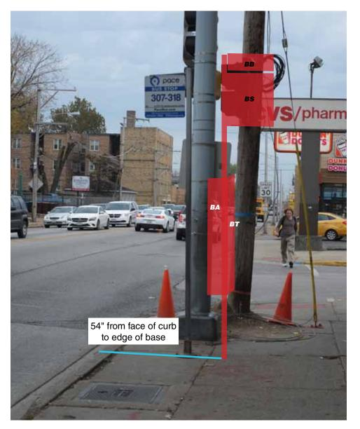
New sign panels, cabinets, and base replace existing sign post and base. Position sign base so anchors do not hit concrete seams.
