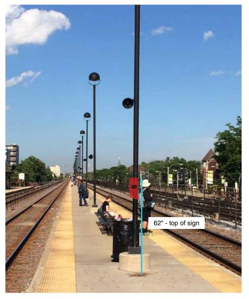
New sign panel mounts to existing light post. Located on second light post east of entrance. Coordinate mounting with OP1-051-S.
