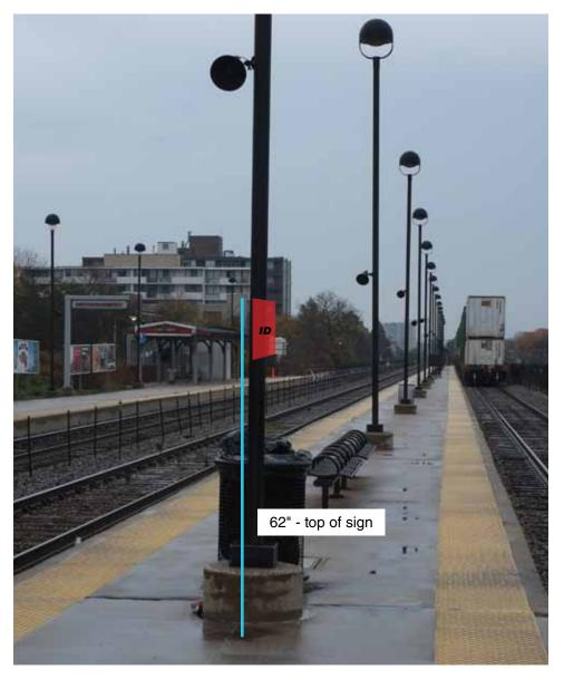
New sign panel mounts to existing light post. Located on second light post east of entrance. Coordinate mounting with OP1-050-N.
