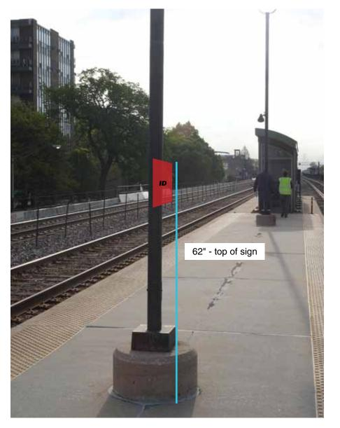
New sign panel mounts to existing light post. Located on second light post west of entrance. Coordinate mounting with OP1-053-N.
