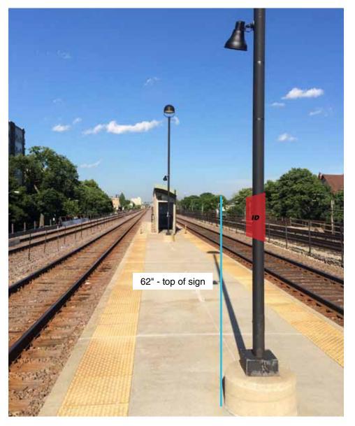
New sign panel mounts to existing light post. Located on second light post west of entrance. Coordinate mounting with OP1-054-S.
