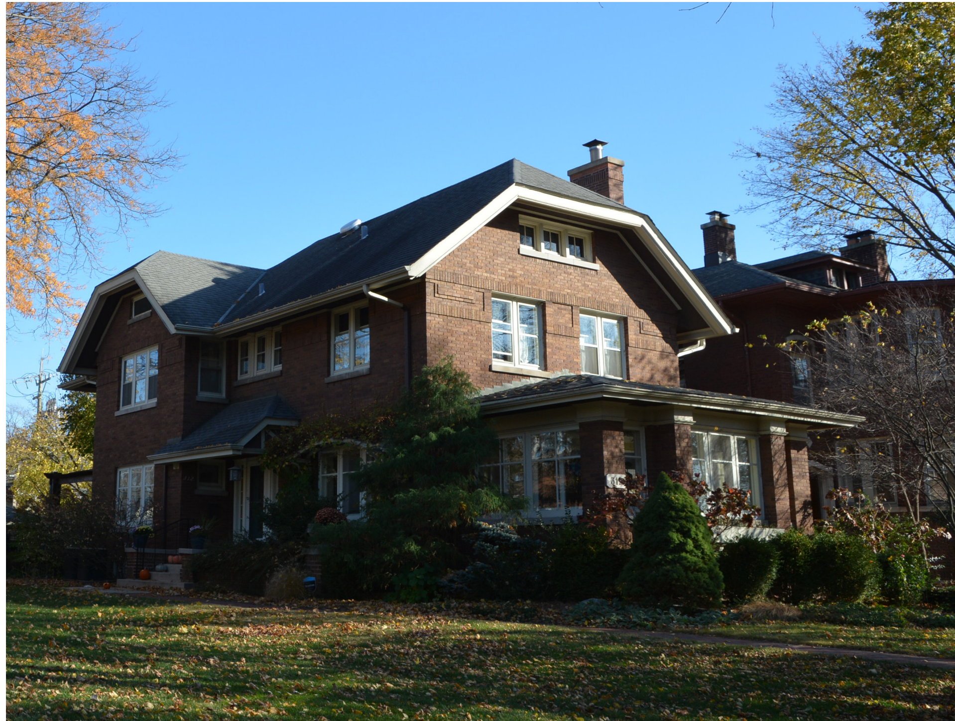
EXISTING RESIDENCE NORTH & WEST FACADES
