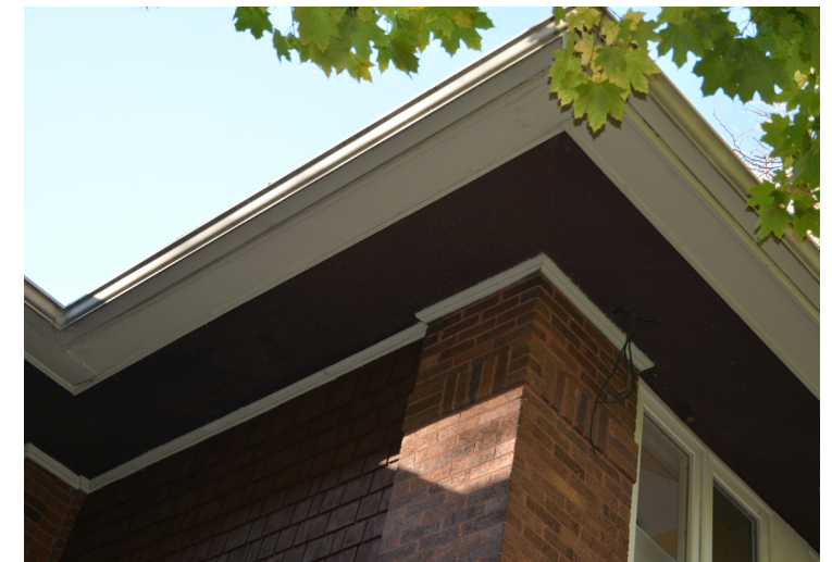
ENLARGED PHOTO OF EXISTING PAINTED CEDAR SHINGLES
