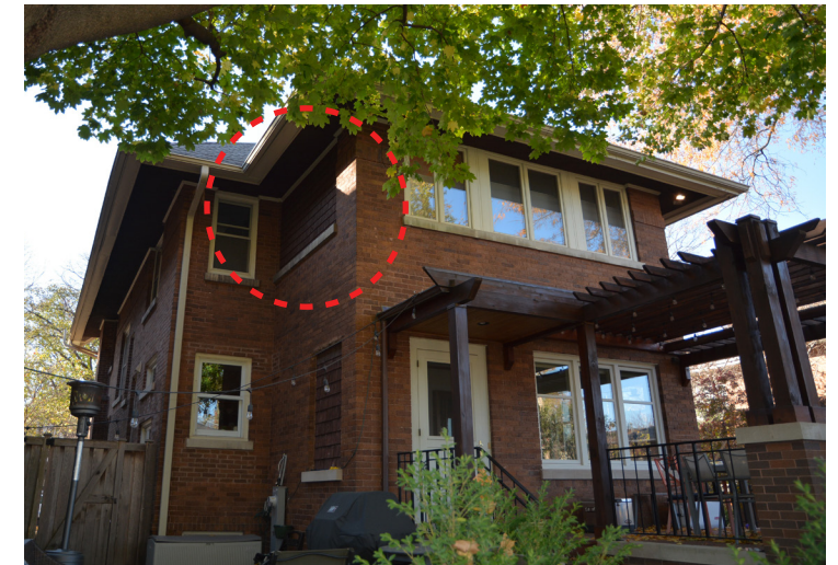
PHOTO OF EXISTING PAINTED CEDAR SHINGLES ON REAR, NORTH SIDE OF RESIDENCE
