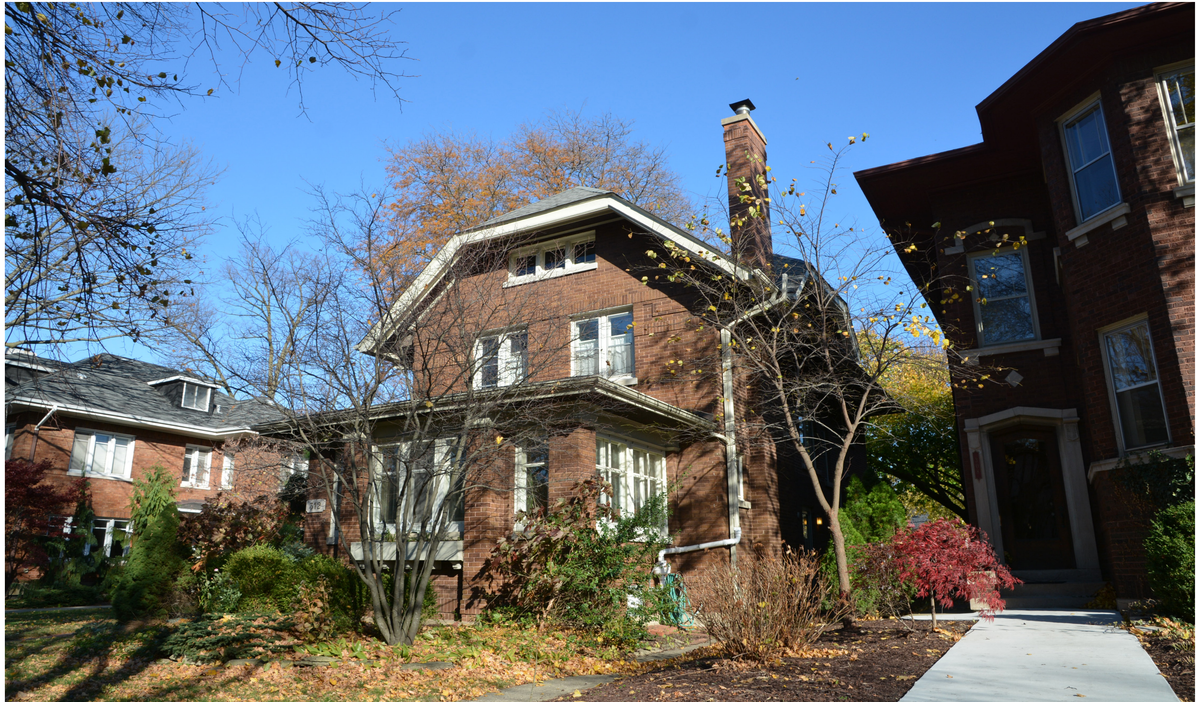
EXISTING RESIDENCE SOUTH & WEST FACADES
