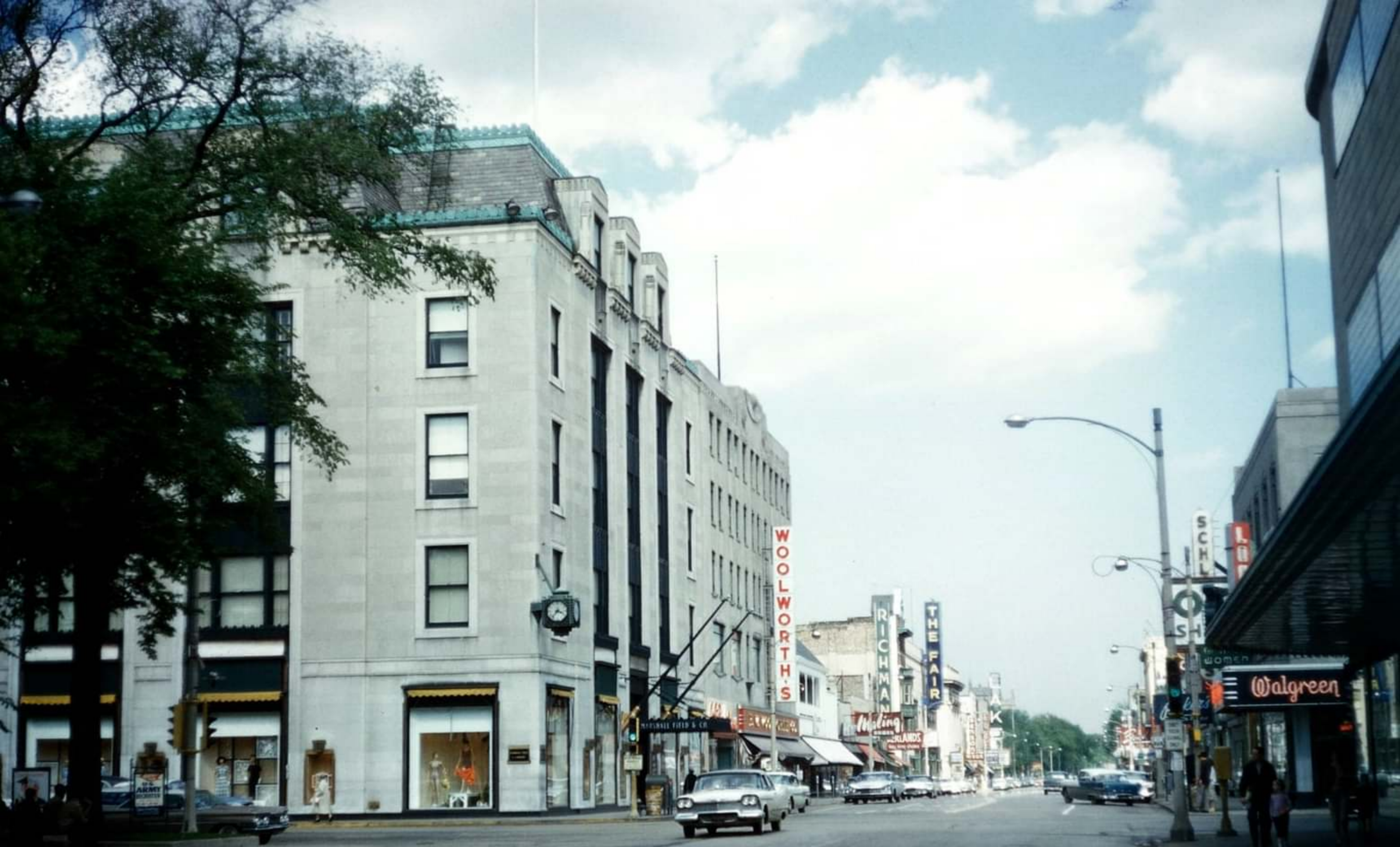
1960 Lake Street - East
