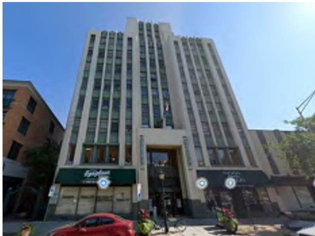
4. LOOKING SOUTH TO 715 LAKE STREET
