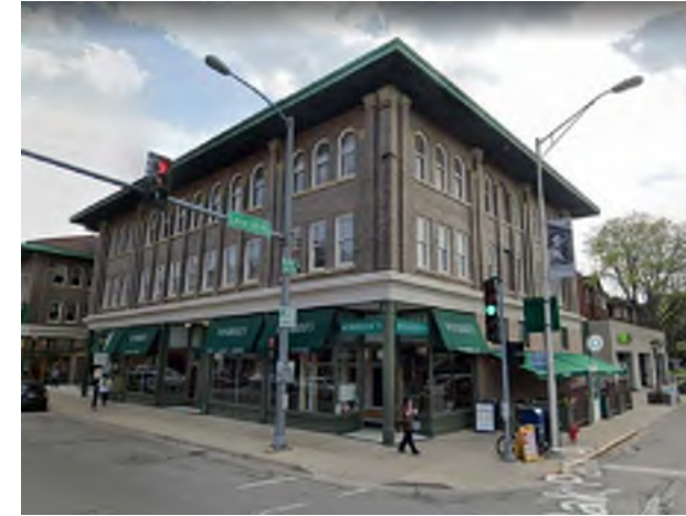
3. LOOKING SOUTH TO 800 LAKE STREET
