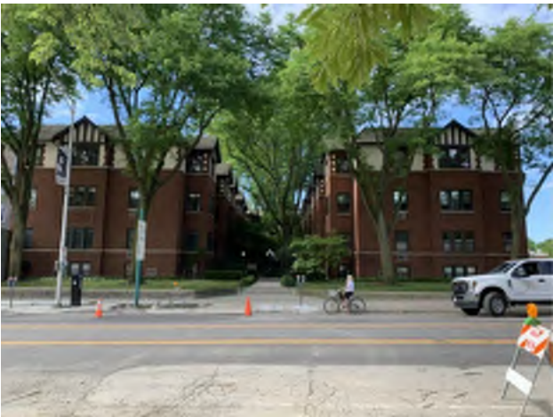
5. LOOKING SOUTH TO 815 LAKE STREET
