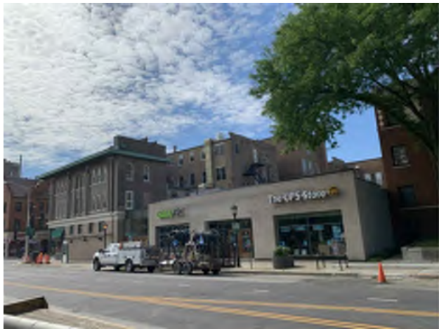
4. LOOKING SOUTH TO 803-05 LAKE STREET
