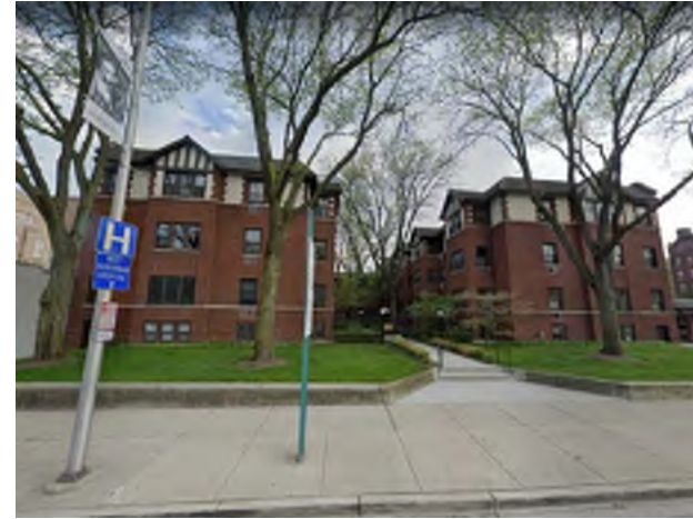
2. LOOKING SOUTH TO 815 LAKE STREET
