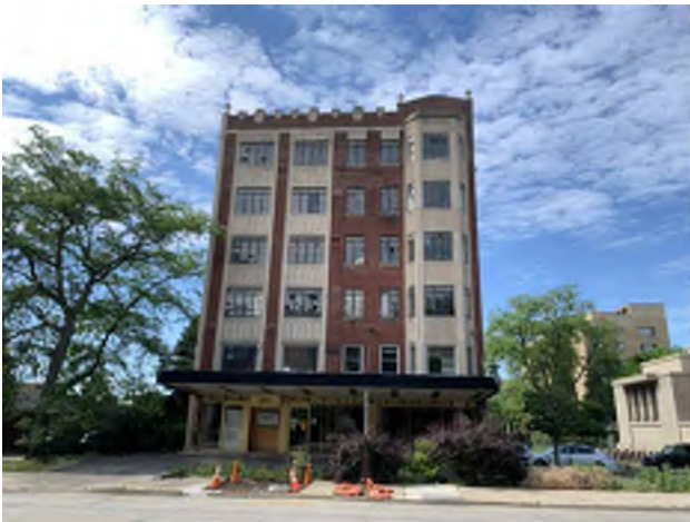
6. LOOKING SOUTH TO 855 LAKE STREET
