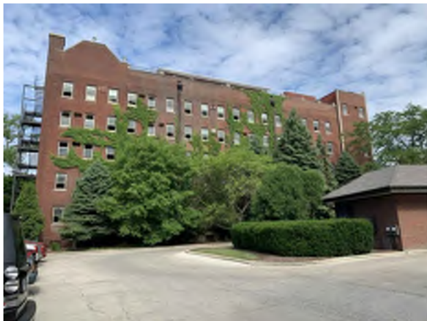
1. VIEW WEST FROM SITE TO 855 LAKE
