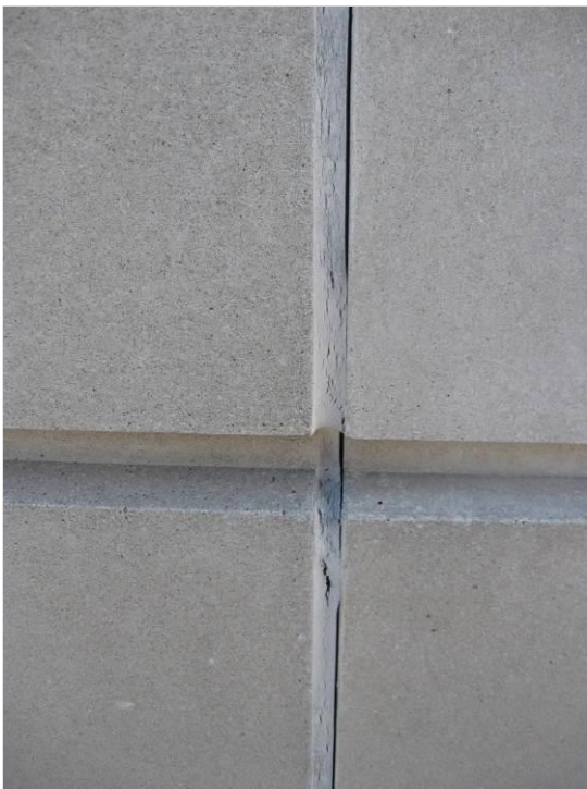
Photo 8 – Severely deteriorated vertical joint sealant on façade panel.
