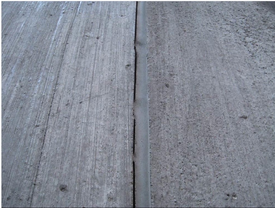
Photo 1 – Adhesion failure of tee-to-tee joint sealant.
