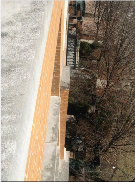
Photo 13 – Broken cap stone with the potential to fall off, south elevation.
