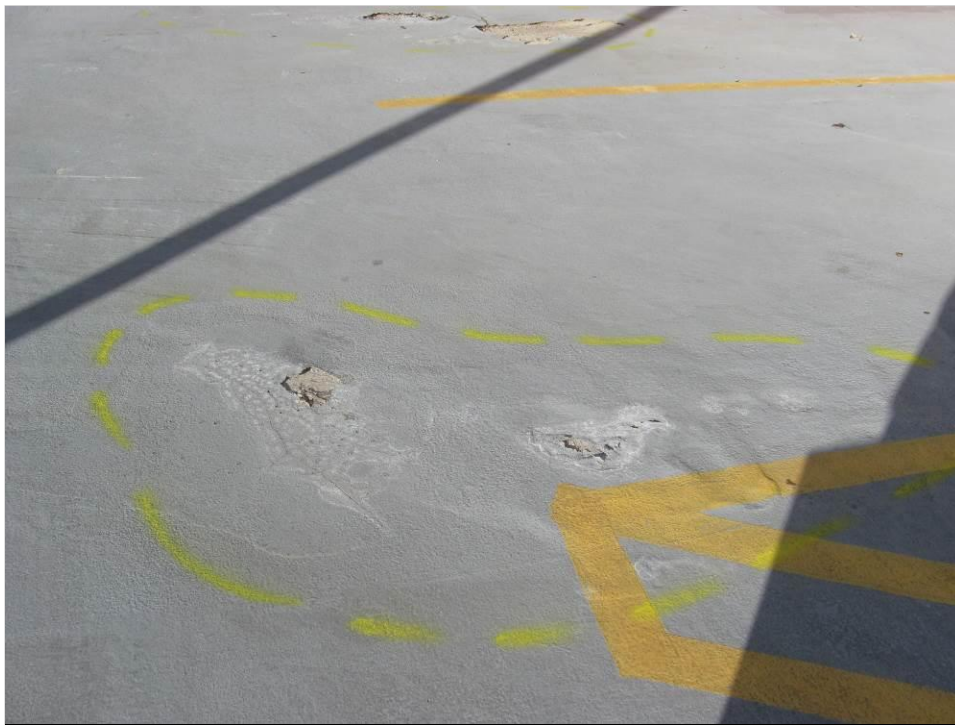
Photo 2 – Concrete deterioration in floor slab under traffic topping.
