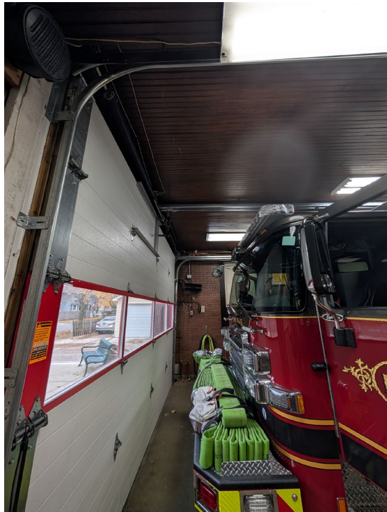
INSUFFICIENT CLEARANCES AROUND ENGINE / NO ROOM FOR ADDITIONAL VEHICLES
