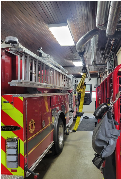
INSUFFICIENT CLEARANCES AROUND ENGINE / NO ROOM FOR ADDITIONAL VEHICLES
