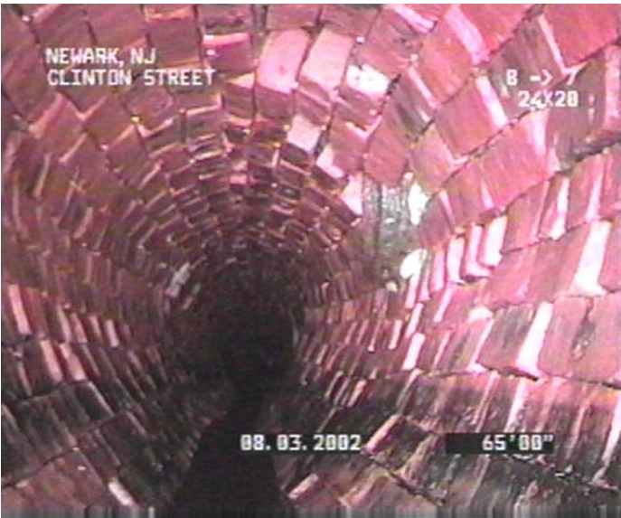
Figure 3. Example of Condition Grade 3 Brick Sewer Collapse Unlikely in Immediate Future; Further Deterioration Likely
