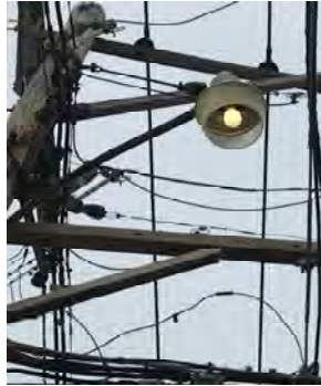
100W Mercury Vapor Alley Light Fixture
