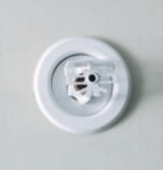
Sidewall Sprinkler
