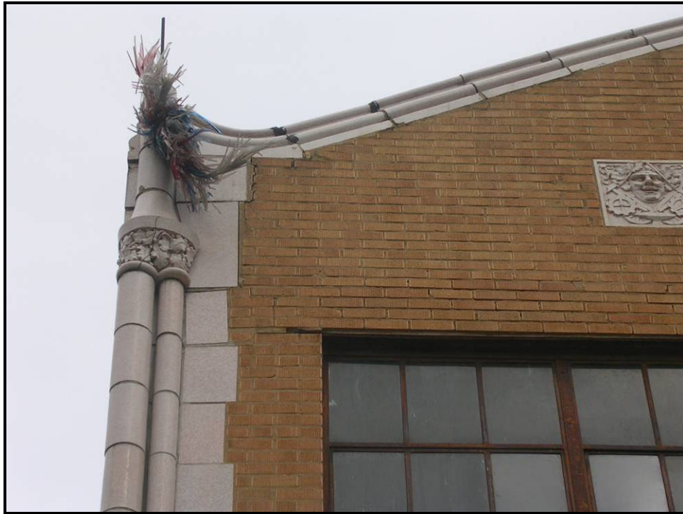
Figure IV – 5: Terra Cotta Quoining on the top Out of plumb with the rest of the building
