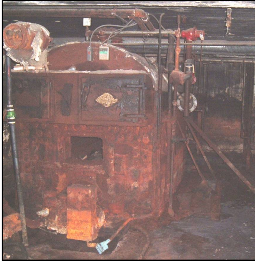
Figure III - 30: Wa-Tu-Bo Boiler
