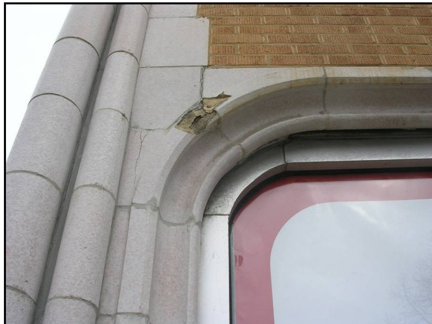
Figure IV - 4: Cracked Terra-Cotta At corner of display window
