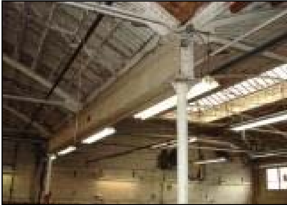
Figure III-20: Steel frame construction of East service area
