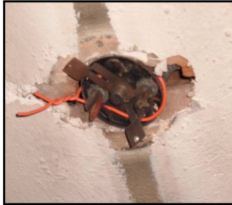
Figure III - 45: original overhead light connection
