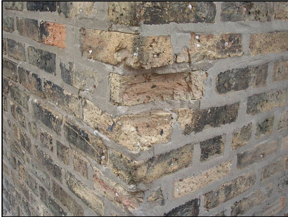
Figure IV – 3 – North Façade Crumbling brick due to impact
