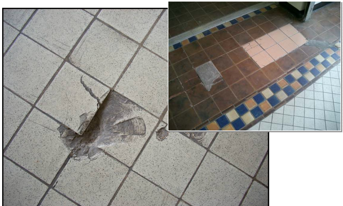
Figure IV – 12: Impact damage & Inappropriate Repair & Replacement
