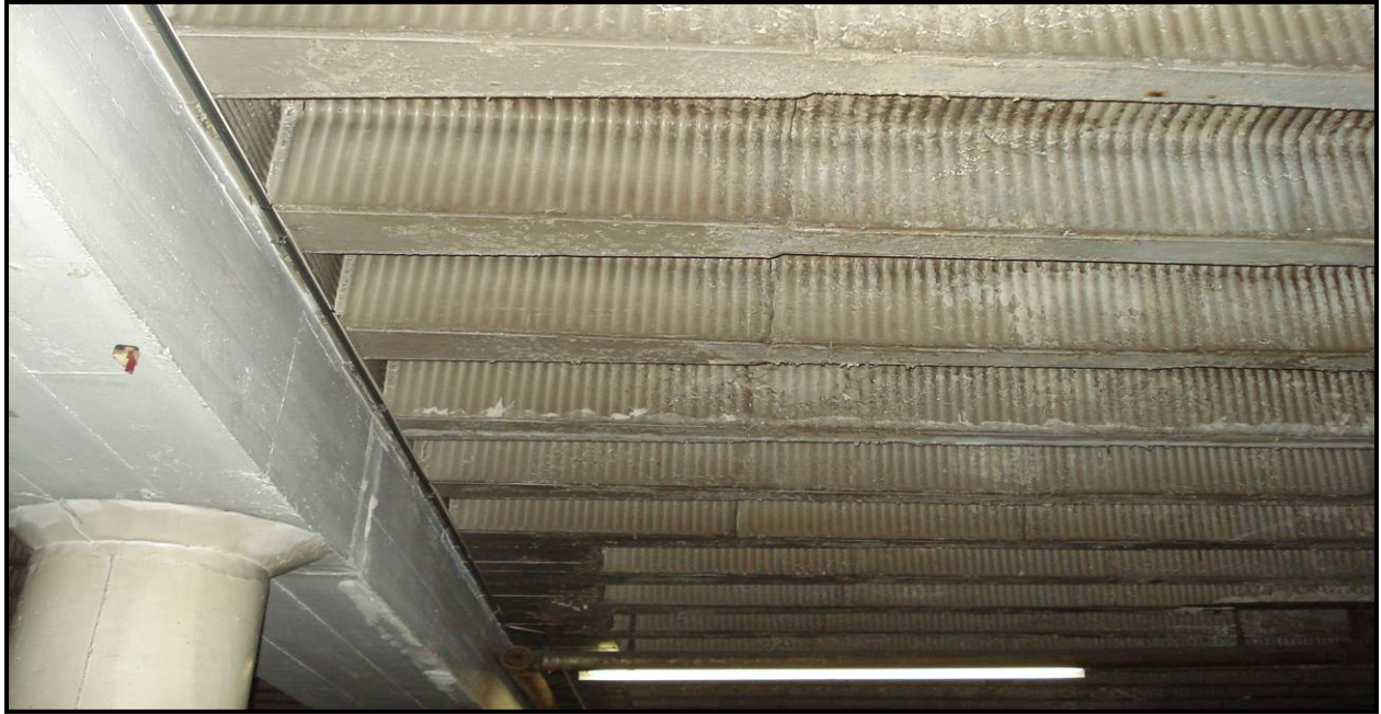
Figure IV- 15: Bowed concrete support beam in West service area.
