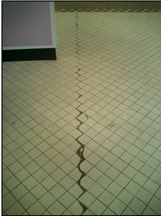
Figure IV – 11: Continuous cracking
