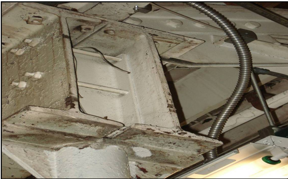
Figure III - 21: Bolted steel trusses and steel columns, welded seat plates
