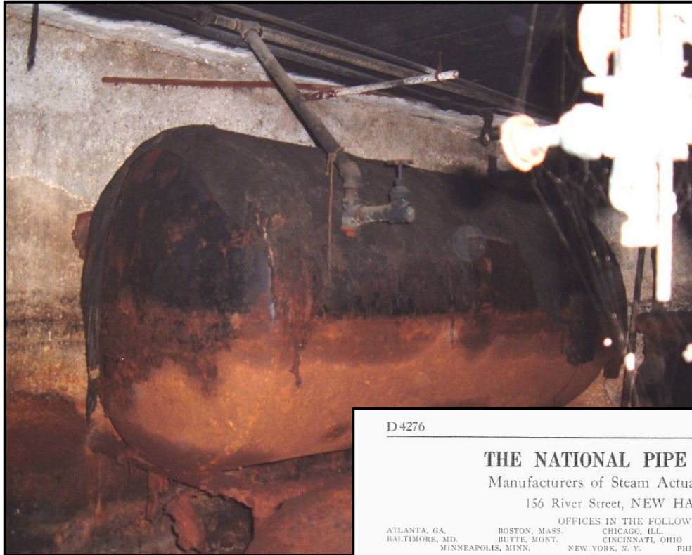
Figure III – 32: Hot Water Storage Tank
