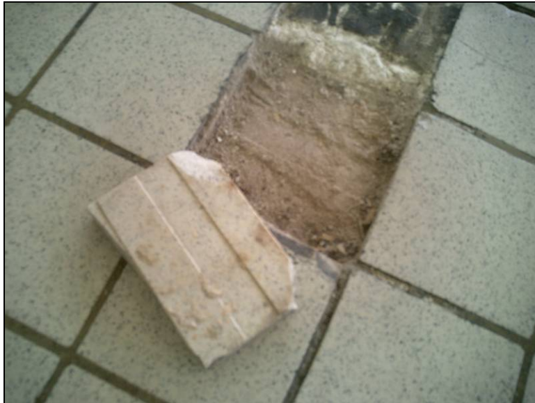
Figure IV – 10: Cracked tile
