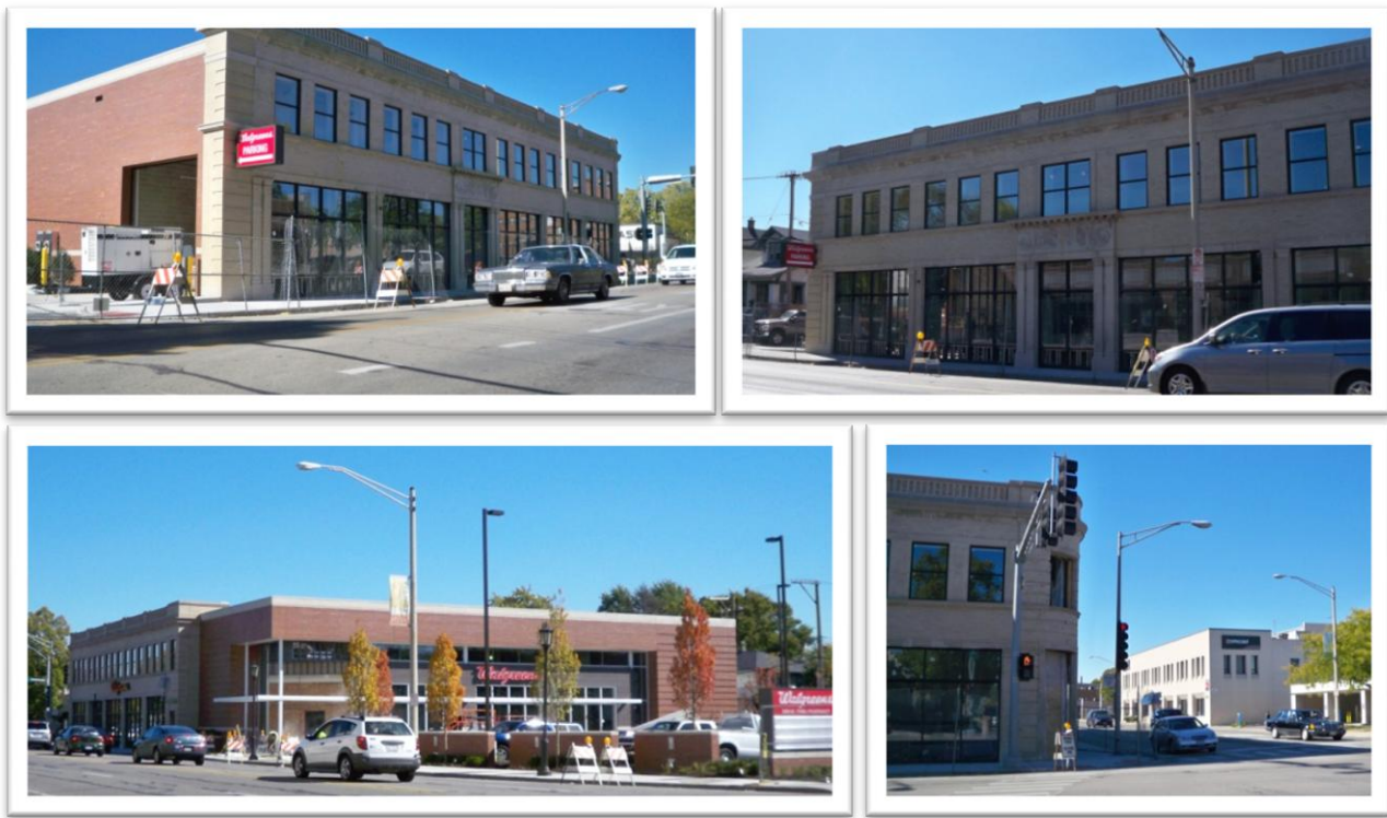
Figure 15, 16, 17, 18- Walgreen’s drug store “Façade-etomy” - where the original Collins building façade was saved and the new “green” Walgreen’s was built behind the façade. Red brick along with brown Dryvit elements are part of the new building; the blond brick is from the historic building.
