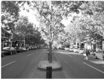
Center medians provide a refuge for pedestrians when crossing the street and narrow drivers' cone of vision, forcing them to slow down.
