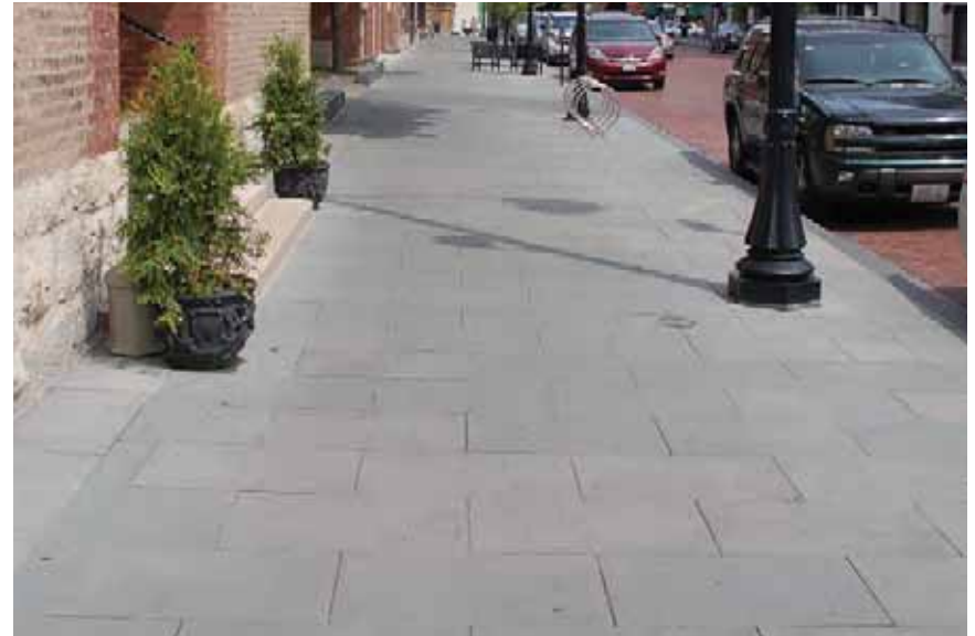
Bluestone Sidewalk: Thermal cut bluestone
