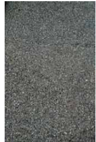
Concrete Curb: Tinted concrete with exposed granite aggregate
