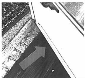
Currently the door only opens a third of the way due to scraping on the boards
