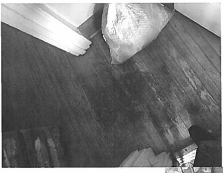
Main path of travel, many nails that were sticking out were removed or countersunk, boards are loose in many areas
