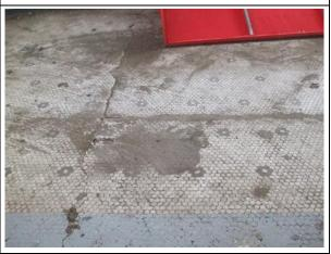
Photo #16 HA 15: Grout and mortar on 1" hexagonal ceramic floor tile (Non-ACM)
