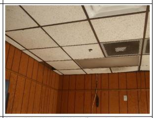
Photo #12 HA 11: 2'x2' hole/fissured ceiling tile (non-ACM)
