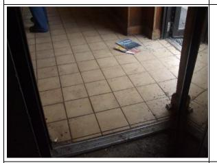
Photo #17 HA 16: Grout and mortar on 8" tan ceramic floor tile (non-ACM)
