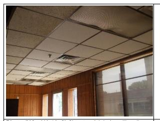
Photo #13 HA 12: 2'x2' texture/pinhole ceiling tile (patch) (Non-ACM)
