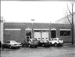
The rear (north) facades are simple brick walls with window and door openings. The east half is yellow brick with no openings, one metal vent, and a stepped parapet with clay tile
