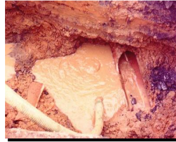
Hidden leak running into drain tile
