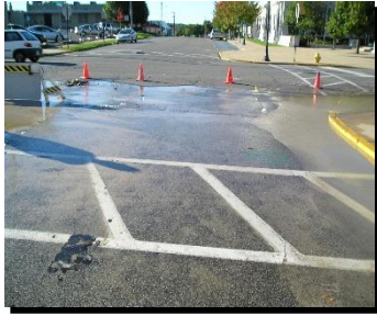
Leak surfacing at intersection
