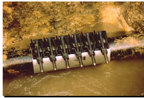
Leak repaired.
