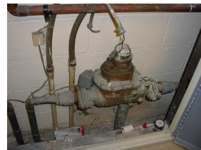
2" Sensus PT meter with remote register
