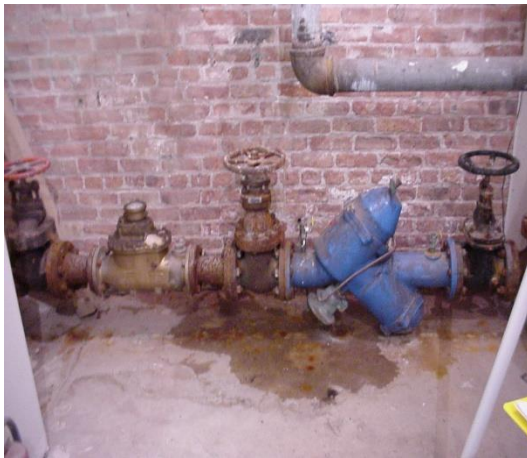
Sensus compound meter with RP2.
