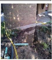
This project involves improving the drainage in the inner parkway area west of the Village Hall geothermal vault. There are three sump pumps and one roof downspout that need to be connected to the existing sewer line that drains into the Madison St. basin.
