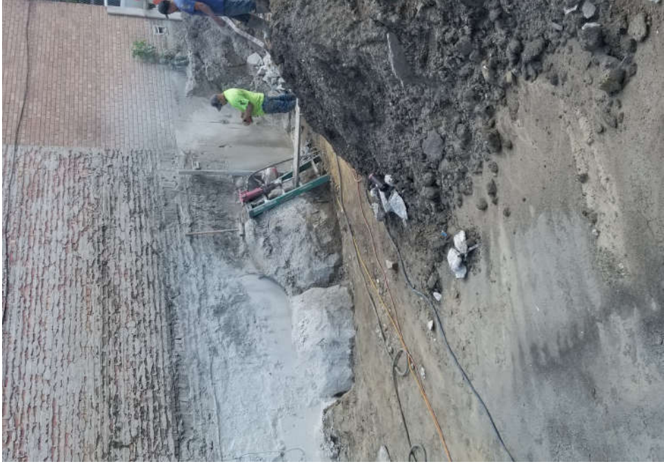
Concrete blow out from neighboring building
