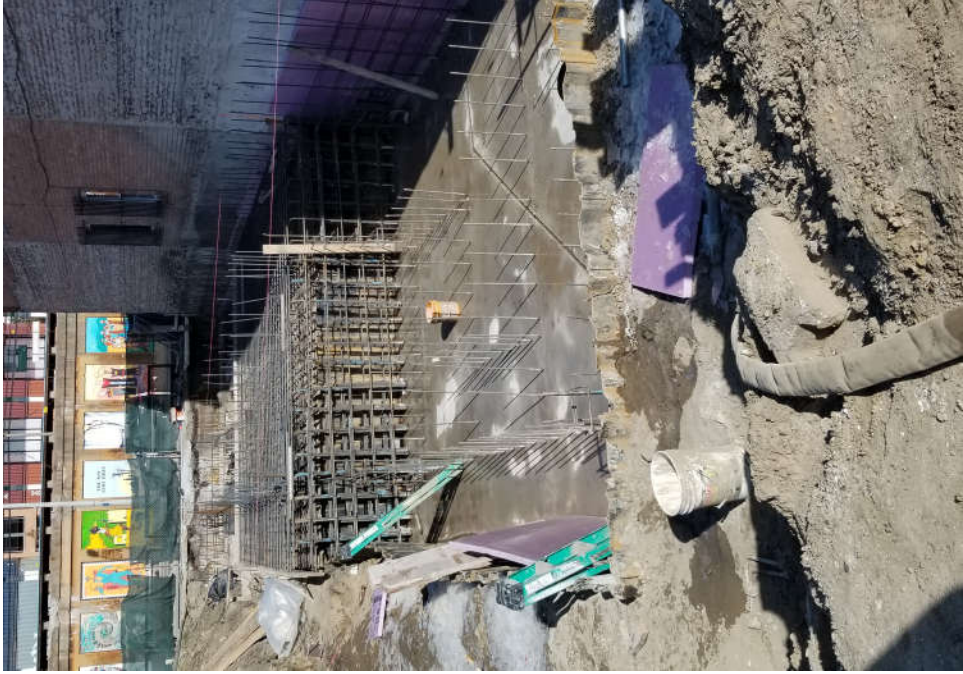
area with lowered foundation, dealing with high ground water level
