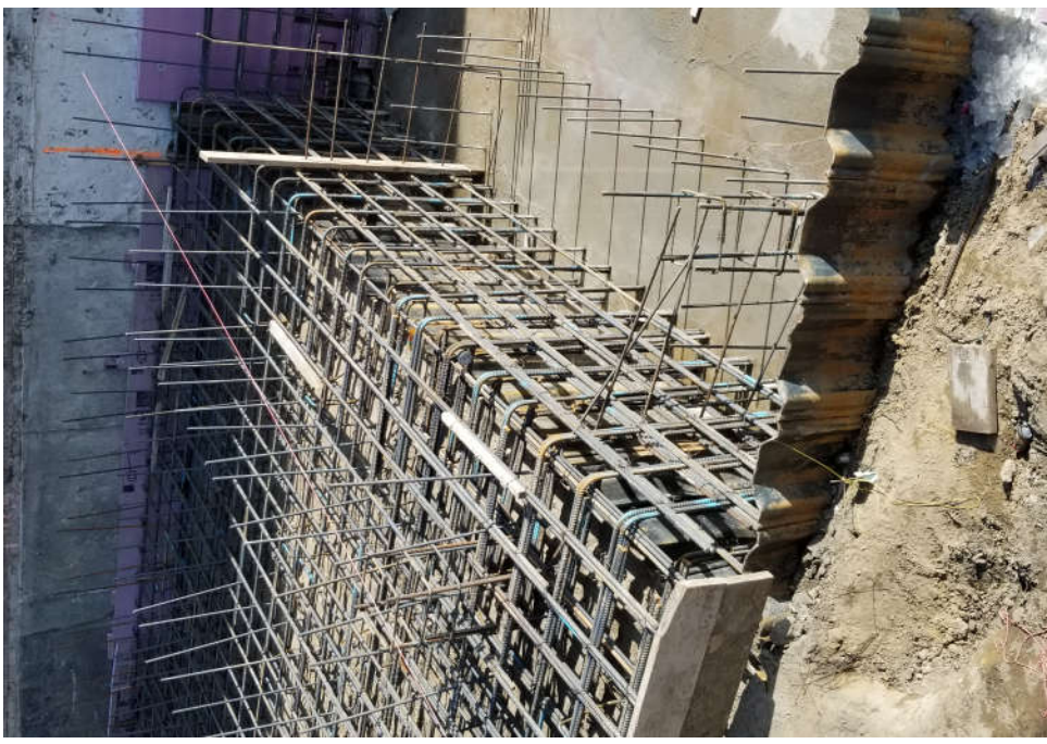
foundation lowered to match neighbor's footing depth, steel sheet piling
