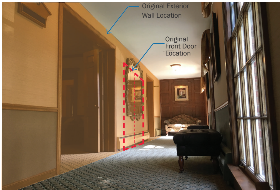
Entry Parlor (in location of original front porch - dashed line indicates approx. location of original front door. Original first floor windows were removed)
